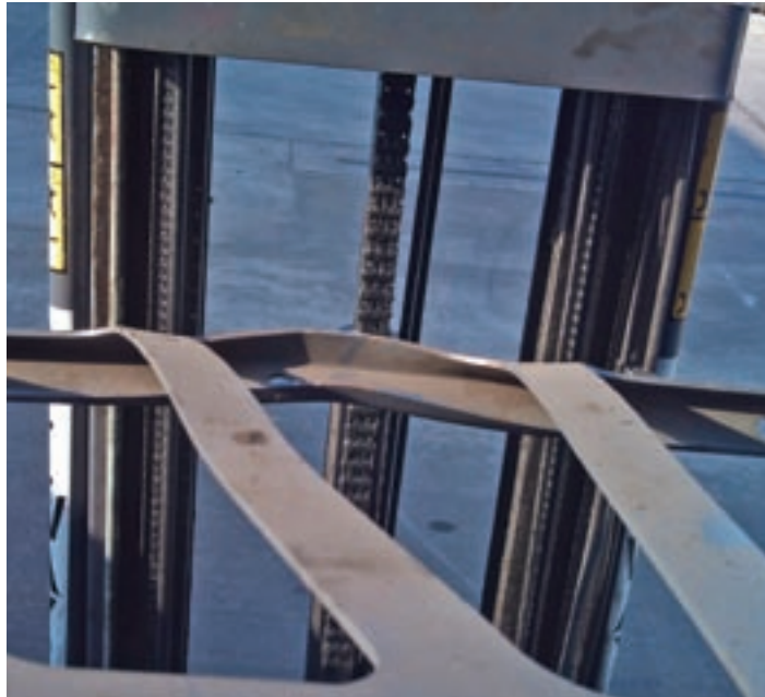
● A chance visit by a service engineer trained to carry out Thorough Examinations under the CFTS national procedure identified severe structural damage that rendered the truck unsafe and unlawful.
