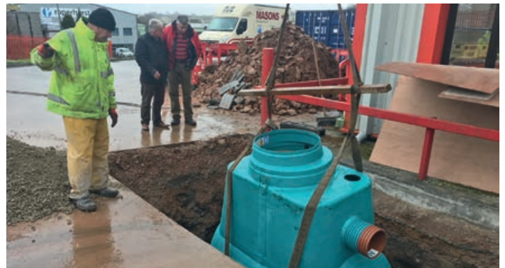
● Gordon Mason overseeing the installation of the interceptor.
